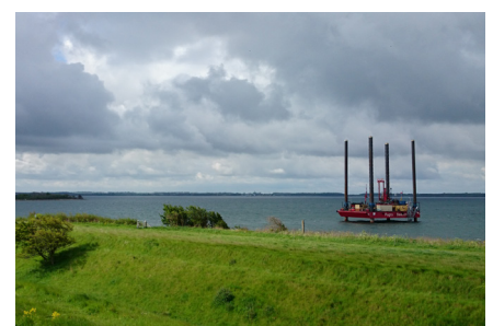
Aran 250 on site in Storstrom, Denmark.
